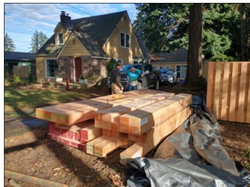
Timbers arrive for the pavilion
