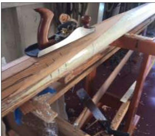
Three-foot long SWALLOWTAIL SCARF JOINT joining new upper mast segment (unpainted and shown planed to 16 sides) to old lower segment.
