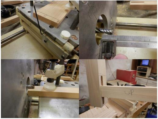
You will be cutting a small piece off of the top and bottom of the apron cheek so it fits into the smaller mortise.
