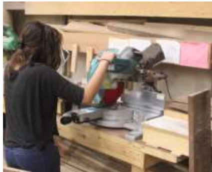
Trimming skirt boards
