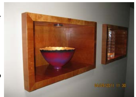
Display cases built through a wall
