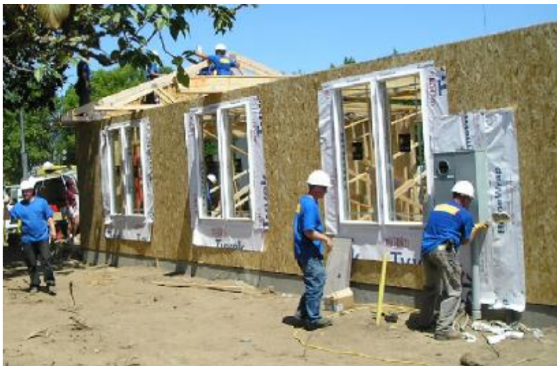
Walls, siding, trusses, roofing, windows, electrical—all at the same time
