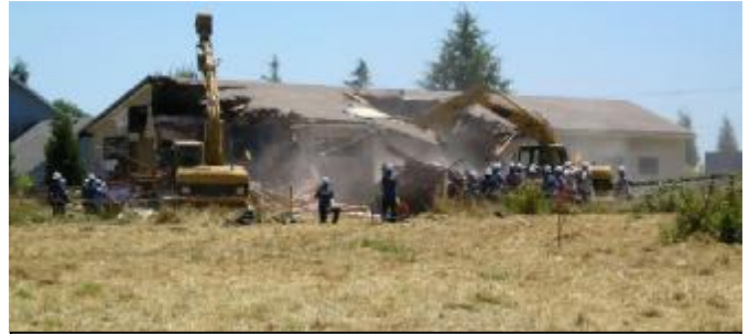
Demolition begins—twenty minutes work
